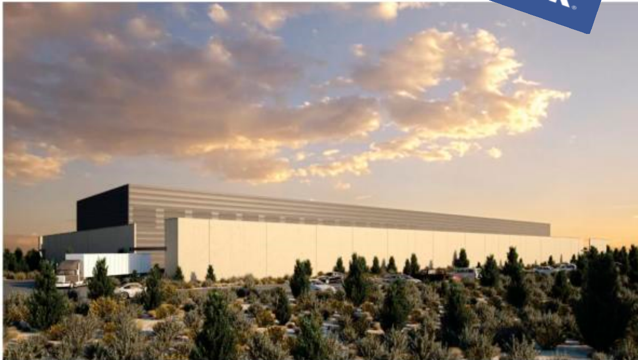
facebook data center in Oregon
